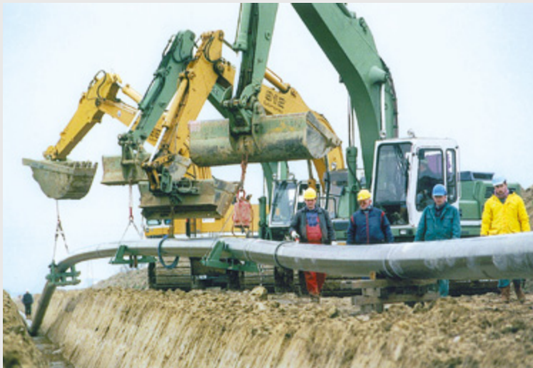
Figure 3: Bend radii in a welded pipe string being lowered into the trench
